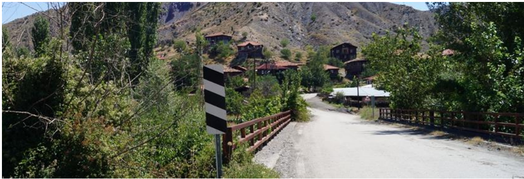
Figure 3.28. Reinforced concrete bridge connecting two sides. (Author, 2020)
