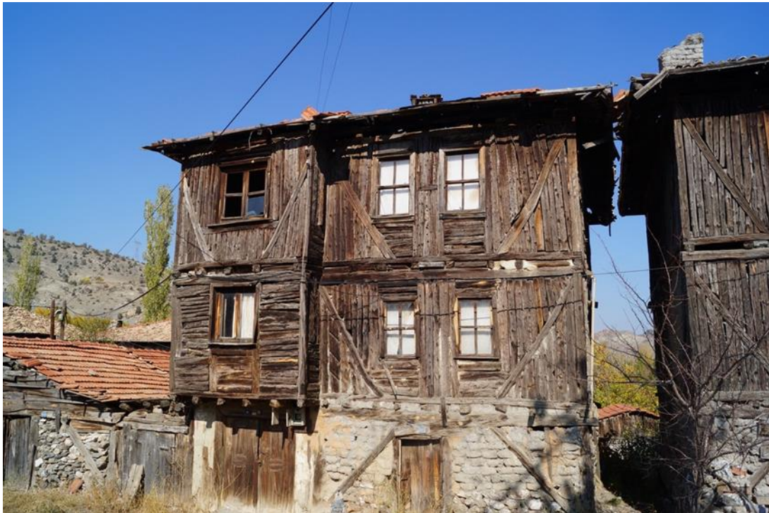
Figure 3.54. Example of 3y3x2c elevation type. (Author, 2021)
