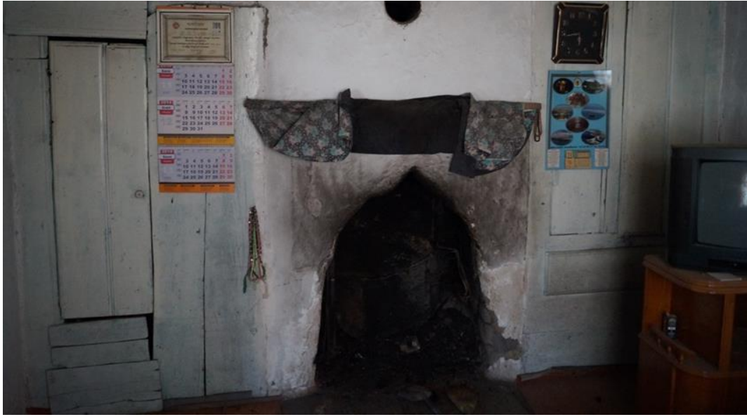
Figure 3.59. Service wall of a room. (Author, 2021)
