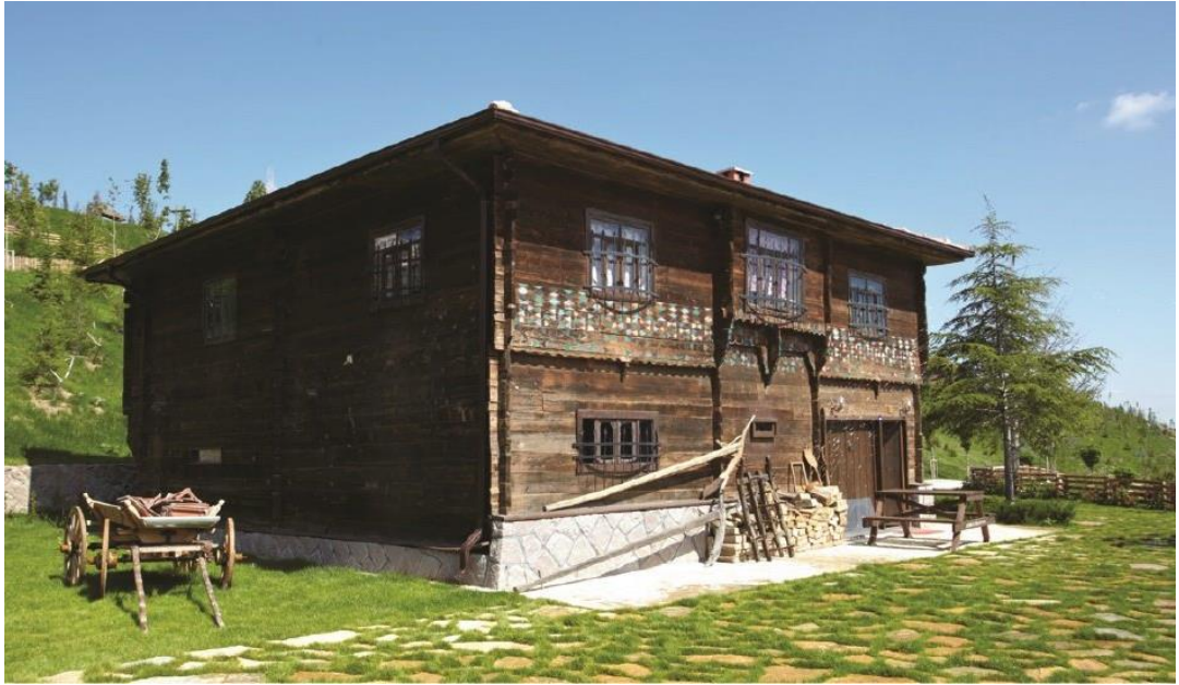
Figure 2.11. Altıncıköy (Altındağ Municipality, n.d.)
