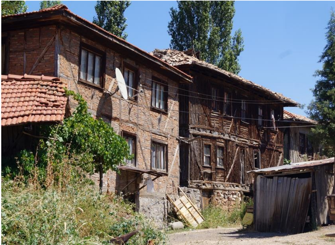
Figure 3.48. Hımış buildings with brick and timber infill. (Author, 2020)
