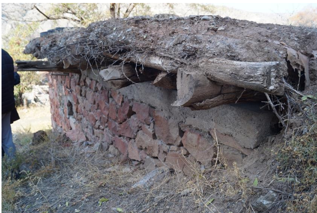
Figure 3.51. Flat roof with mud covering. (Author, 2020)
